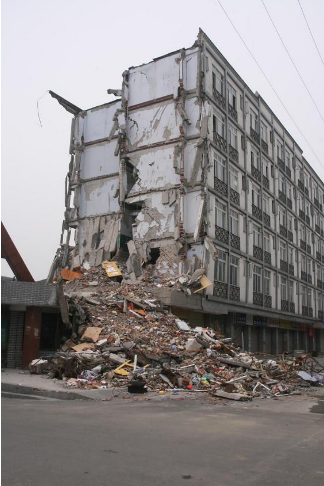
Collapsed building in Dujiangyan
