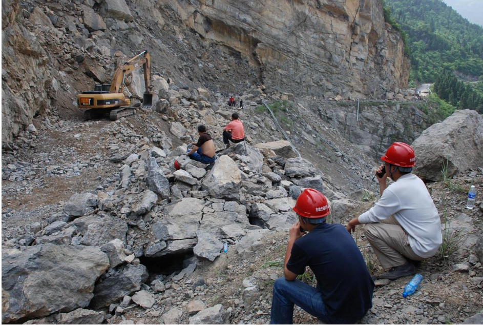
Dangerous and slow process in recovering the damaged mountain highway
