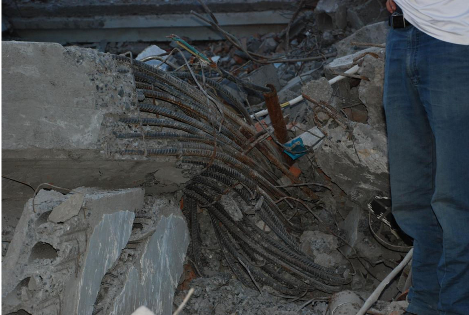
Poor design with too many longitudinal bars but little transverse bars
